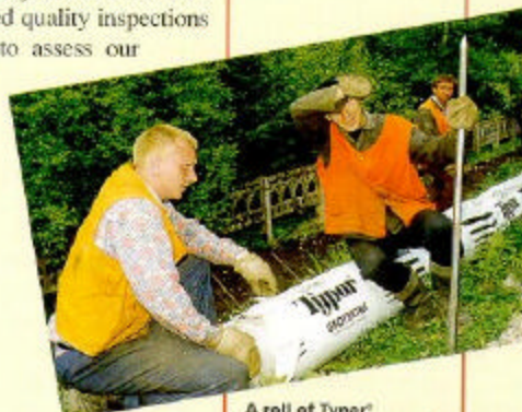
A roll of Typar® geotextile is prepared alongside the railway track.
