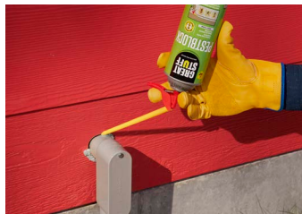
Electrical Cable Lines
